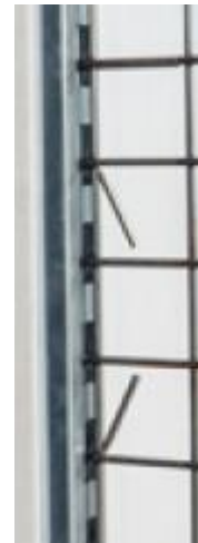
Picture 6. Locking of every 3 rd iron bar for wall classes 2 and 3
