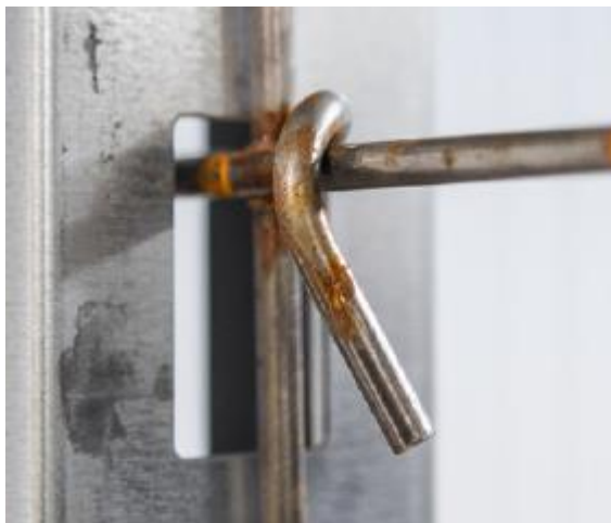
Picture 7. Locking "knot" for every 8 th iron bar for wall class 3.
